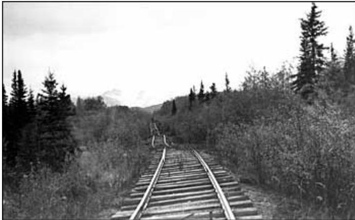
The abandoned Copper River and Northwestern Railway near Strelina in south-central Alaska illustrates how building a railroad on permafrost thaw can cause the railroad bed to settle unevenly. Although maintenance and use of the railroad was halted in 1938, lateral displacement continues today. (Image courtesy of U.S. Geological Survey)
